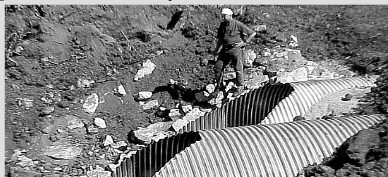
Commissioner Vaughn inspects a new 96" tinhorn near Henney Road.
